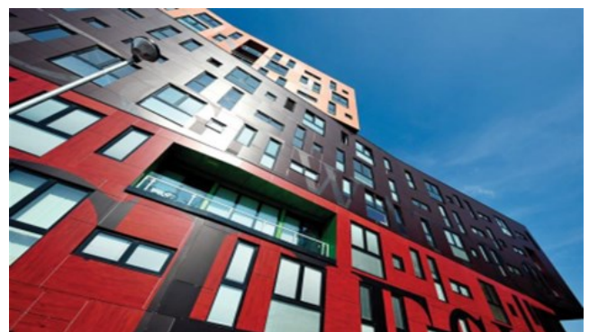
Overcoming the High Rise Challenge in Manchester
