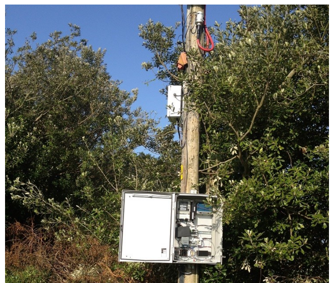
Rugged Modem carries data to the coupler above
