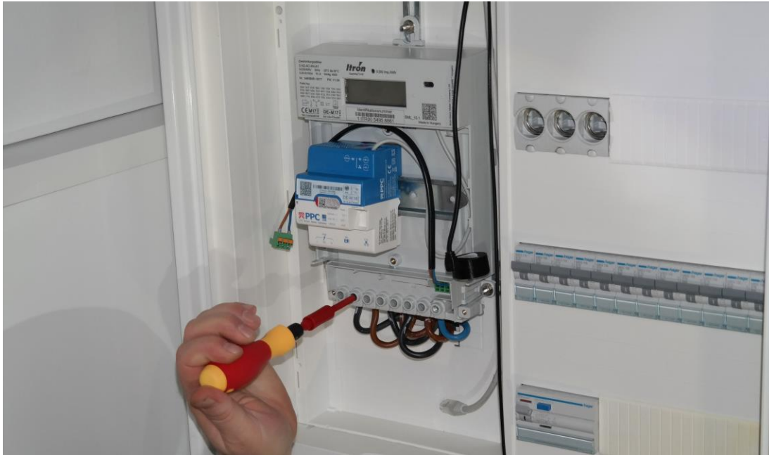
Fig. 3 Installation of the first certified Smart Meter Gateway
